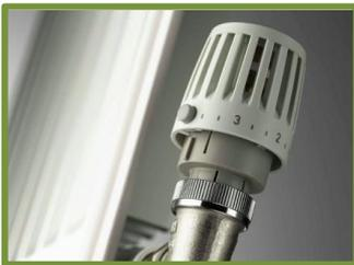
Thermostatic radiator valves can be retrofitted and are relatively cheap to install. Make sure to leave the space around the valve clear for it to be able to measure temperature properly.
