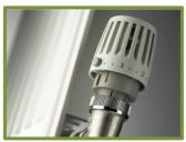
below the set point. So interestingly, they do not work like a tap, there is no proportional control to the flow of hot water. What the 1 to 5 or 6 settings relate to is the air temperature at which the radiator will be turned off. A 1 to 5 thermostatic radiator valve at setting 5 makes the radiator turn off when the adjacent air temperature is roughly 25°C, and at setting 1 it will turn the radiator off at around 15°C.
